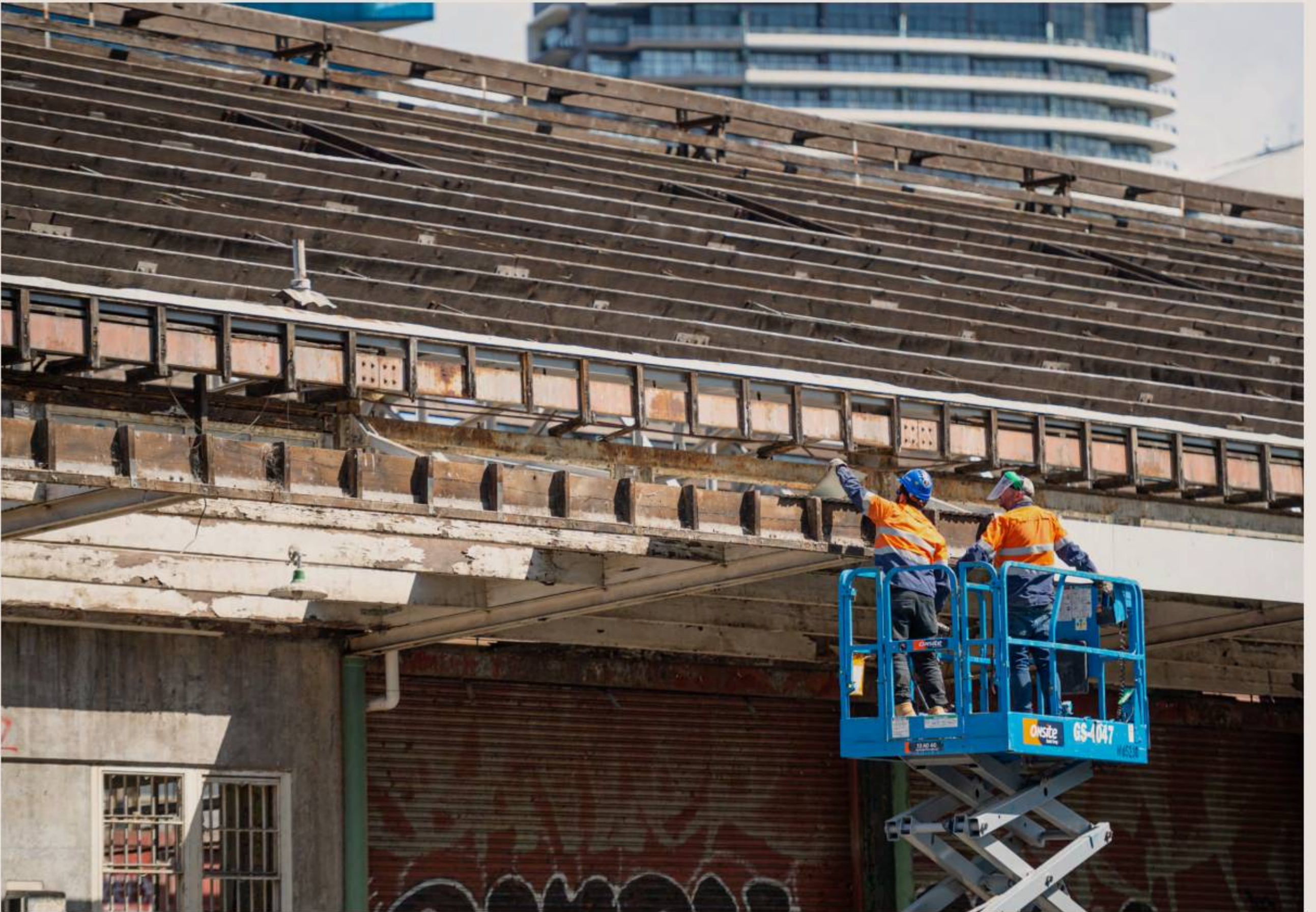
Removal and salvaging of timbers from Goods Shed No.5
